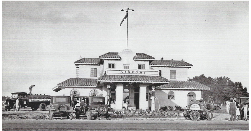
The original 1929 terminal also served as a Standard Oil gasoline filling station. Public domain image provided via the excellent Historic-Memphis.com website.
