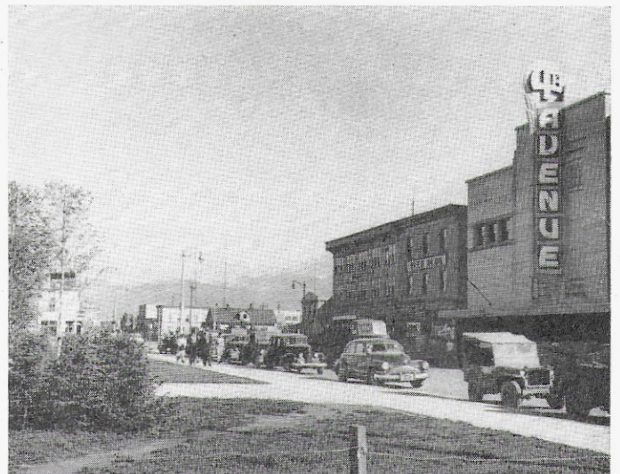
Fourth Avenue, the Main Street of Anchorage
