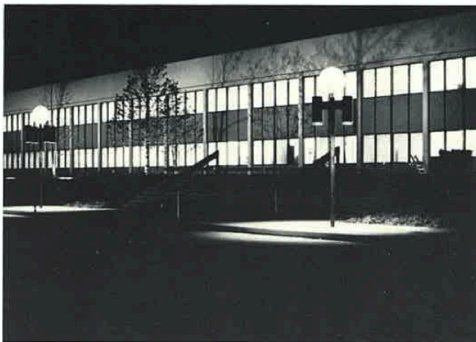
The main entry to North Central's General Office building features a courtyard area, with granite steps and park benches. The area is beautifully landscaped with trees, grass and shrubbery, and illuminated by contemporary boulevard lights.
