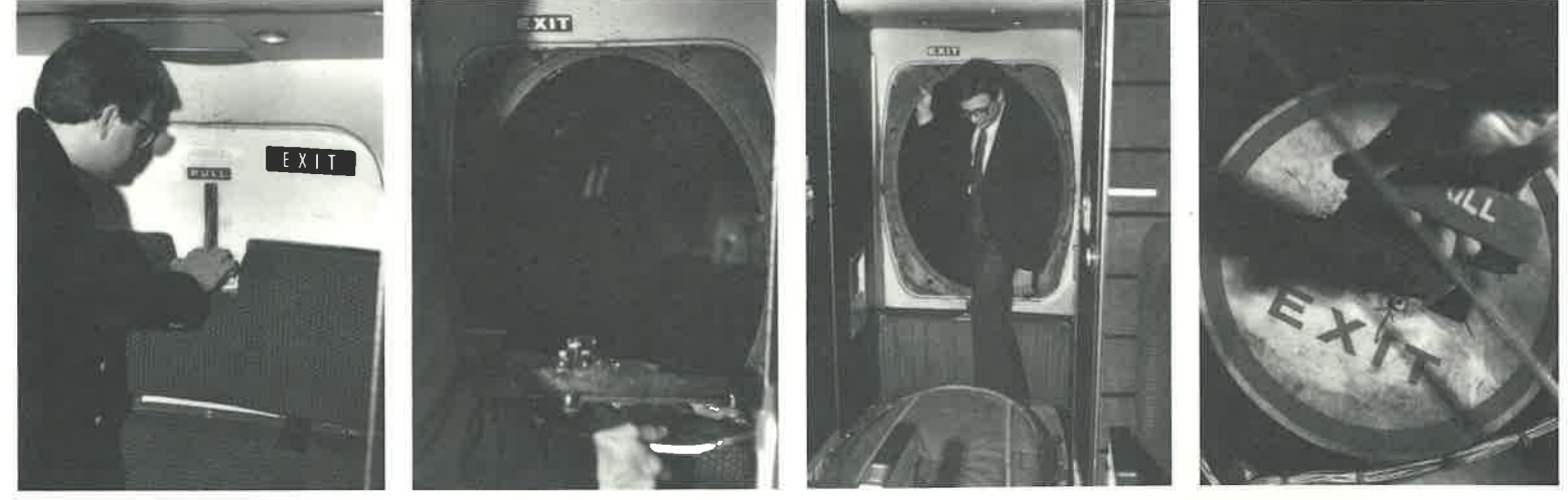
Located at the rear of the aircraft is either a plug hatch type or a pressure bulkhead door. Located in tailcone area.
