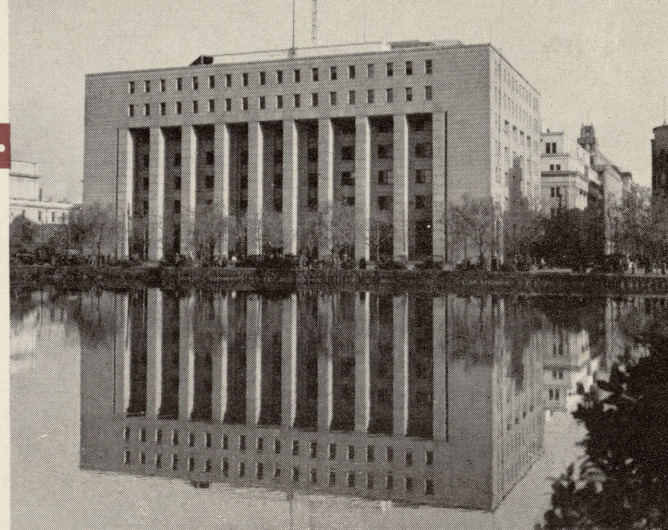
Waters of a moat reflect Dai-Ichi Building, General Douglas MacArthur's headquarters.
