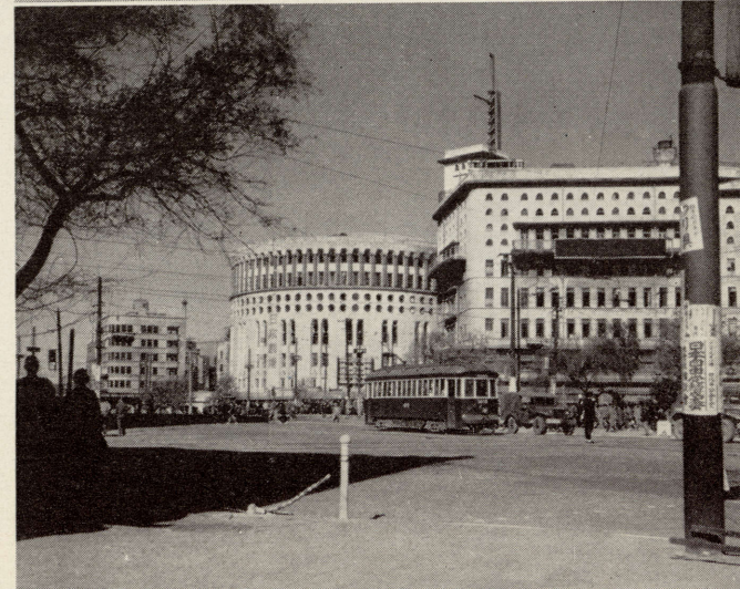
Nippon Gekijo theater, the circular building, adjoins a modern newspaper plant.
