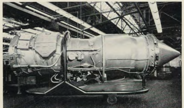
J-75 jet engine ready for final inspection at the Pratt and Whitney factory. The J-75, larger than the J-57, will give Northwest's DC-8s added power and performance.
