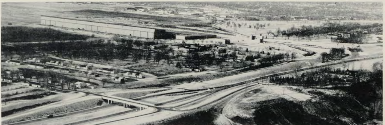
Northwest's system-wide general office and overhaul base, now being constructed at the Minneapolis-St. Paul International Airport, will be the most modern, efficient airline facility in the world. Aerial view shows five overhaul and maintenance hangars which have a total frontage of 1,600 feet—more than five football fields. Finished structure, with more than 1,000,000 square feet of floor area, will be largest in entire Upper Midwest region.
