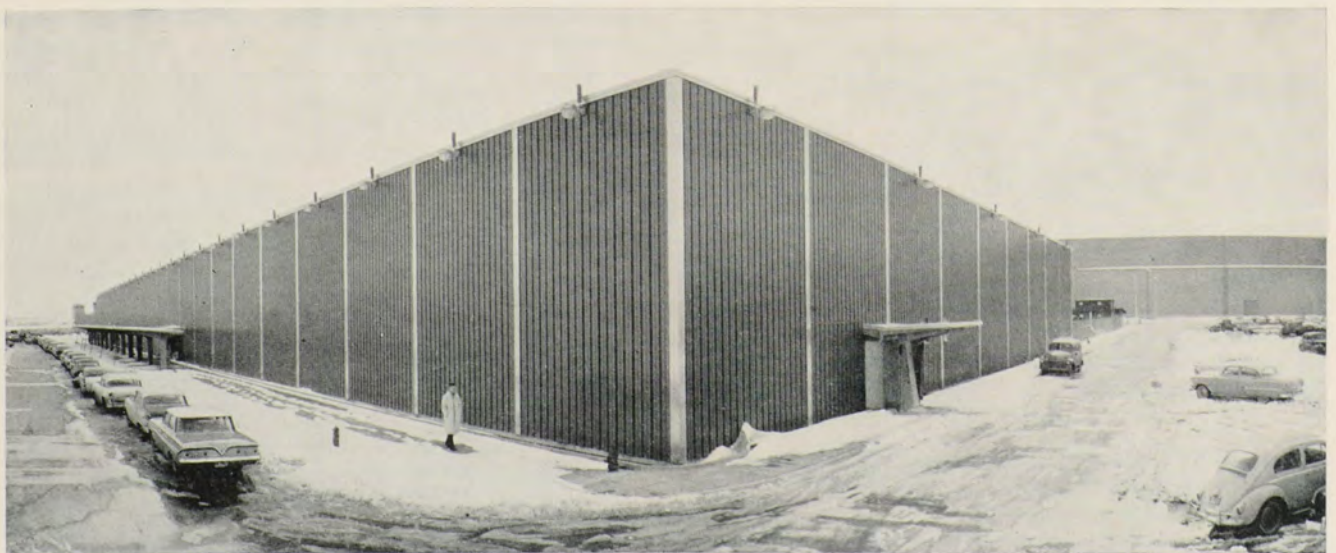
Construction of Northwest Orient Airlines' new General Office building is nearing completion, as part of the Main Base at Minneapolis-St. Paul International Airport. Design of the 259,200 square-foot building is a departure from conventional office design, in that there are no windows in the 33 foot-high exterior panels of blue-green, porcelainized aluminum. The building will be completely air-conditioned. It adjoins hangars (right, background) via shops and stores buildings.
