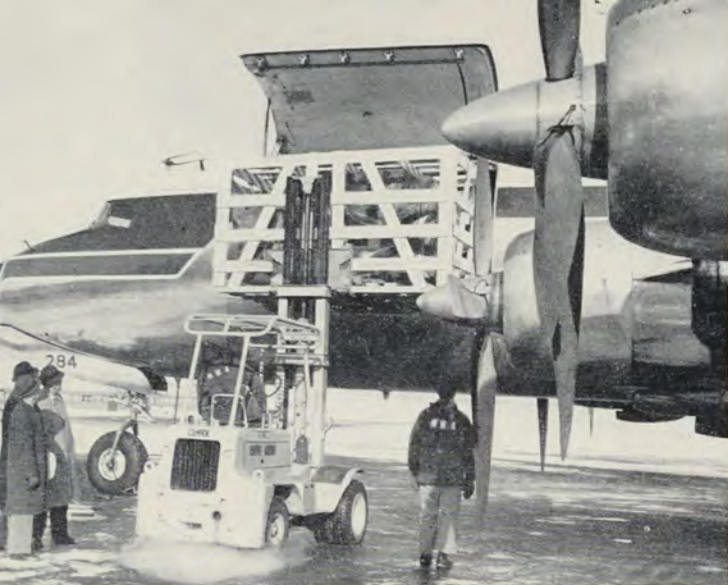
Conversion of five of Northwest Orient Airlines' DC-7C's to freighter configuration, including installation of an 81 by 124-inch forward cargo door, facilitated an increase in freight lift. Piece of paper-making machinery (left), boarded at Milwaukee en route to Gothenburg, Sweden, taxed every available inch of the huge doorway.
