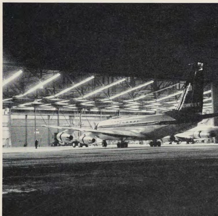
One of Northwest Orient Airlines' Boeing 720B fan-jet airliners is towed into a Main Base hangar at Minneapolis-St. Paul International Airport for routine work. Hangar is one of five at the Main Base, each 320 feet wide and 160 feet deep. Each hangar will accommodate two huge jets or three of Northwest's propeller-driven aircraft.
