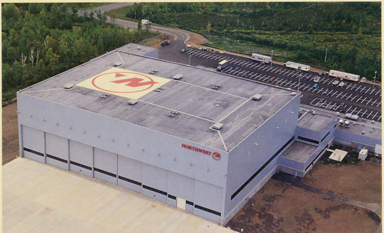
Aerial view of the new maintenance base in Duluth, MN, opened in October 1996, employing up to 350 mechanics.
