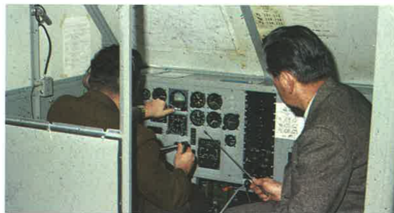
Transdyne navigational trainer permits demonstration of instrument flight procedures.
