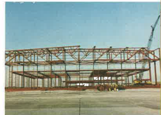
Construction is on schedule.
