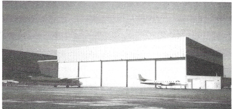
Mesaba's new hangar accomodates more than twice the number of aircraft than the regional airline's former facility.
