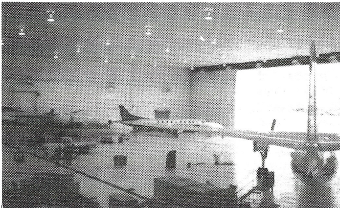
The new hangar measures 225 feet by 229 feet and is 63 feet high.
