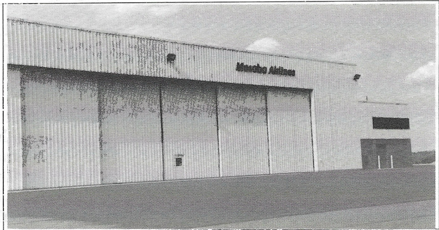
Mesaba purchased this aircraft hangar at Central Wisconsin Airport in Mosinee, Wisconsin. The building features 38,000 square foot of space. Mesaba currently overnights aircraft in the hangar.
