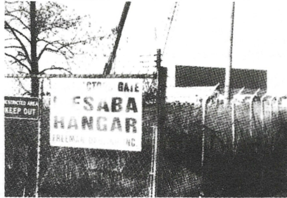
The new hangar looms in the background. It is one of the first major hangars built at Detroit Metro in some time.
