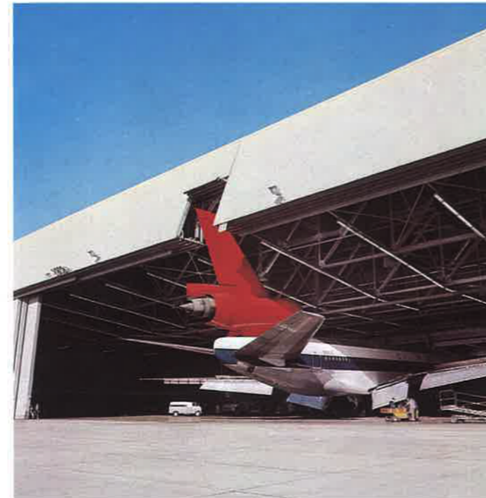
The 'keyhole' cut into existing hangars made room for DC 10-40 jets to be maintained.
