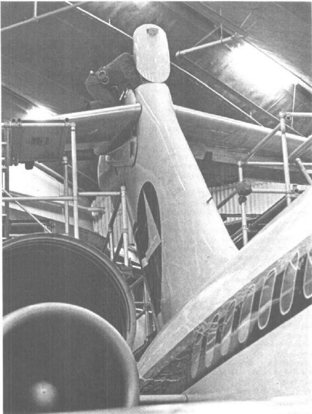
The actuator unit he is inspecting is about 28 feet above the hangar floor
