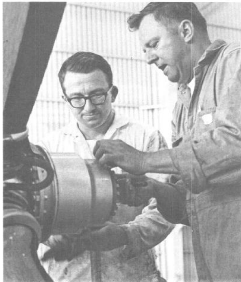
Loren Corlsen and Rudy Mayo rigging a propeller
