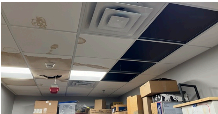
The area behind the checkout counter was soaked and dirty with ceiling tile grit. In the storage room (below), many tiles had already been removed, but the fire alarm dangled where it punched through a waterlogged piece.
