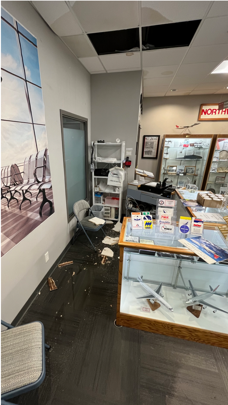
The area behind the checkout counter was soaked and dirty with ceiling tile grit. In the storage room (below), many tiles had already been removed, but the fire alarm dangled where it punched through a waterlogged piece.
